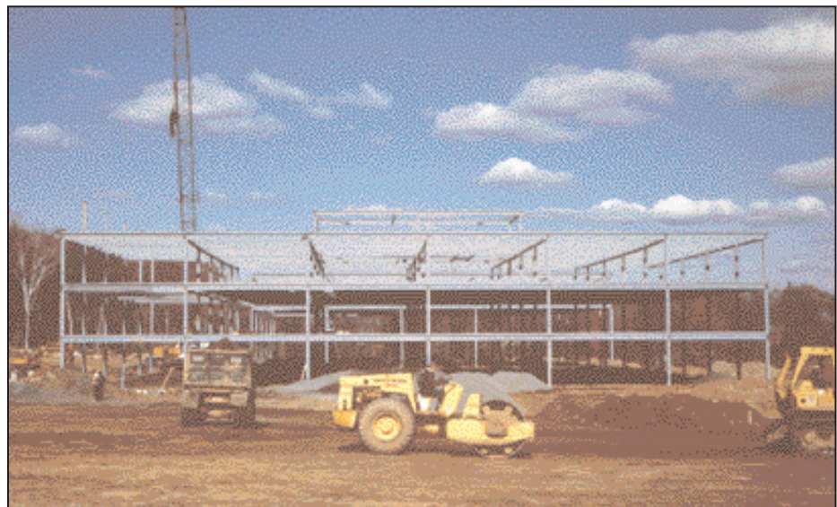
Three-story office facility under construction as the superstructure is set in place.
